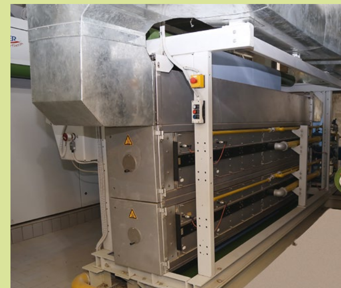
Infrared radiation dryer in operation
