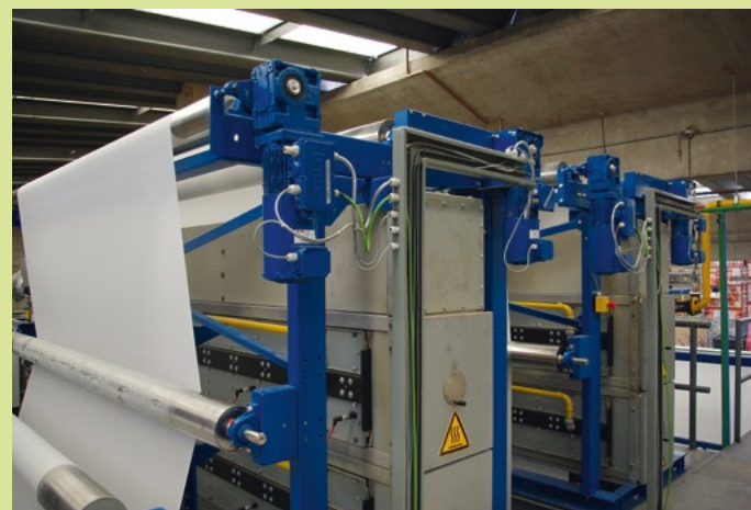
Infrared radiation dryer in front of the stenter
