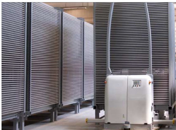
Intermediate storage and automated transport
