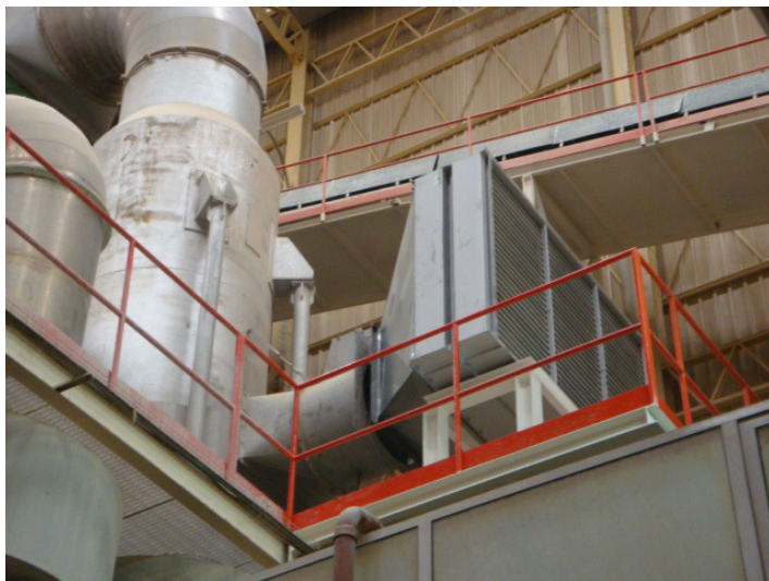
Spray Dryer: Heat Exchanger Water-Air ; Fresh air is sucked trough the Water-Air heat exchanger and heated to ~120°C
