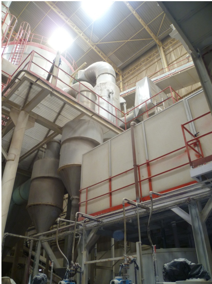
Spray Dryer : General view with Water-Air Heat Exchanger
