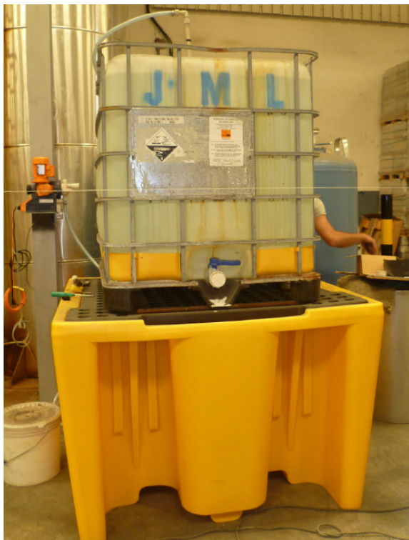
Caustic Soda injection for neutralization of acids
