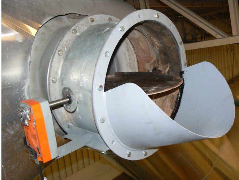
Air-Water Heat Exchanger: Fresh air flap (opens when Kilns on Bypass, or in case of emergency)
