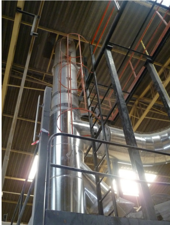
Kiln: Exhaust air burning section ; Connection to chimney, flaps ; Exhaust air to Luwa Heat exchanger
