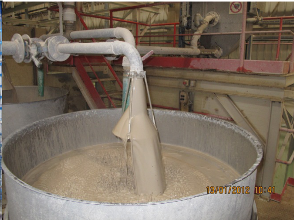
Out of Drum mill: slurried raw material
