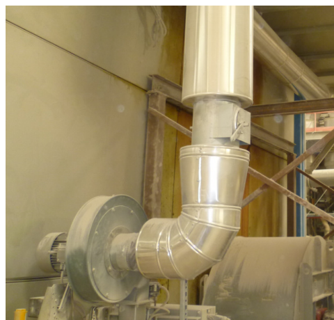
Vertical Dryers: Hot air supply to Burner
