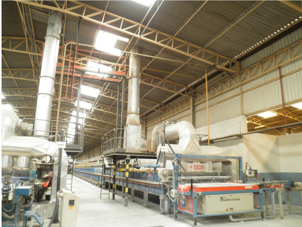
Kiln: Preheating-, Burning- and Cooling Section; Burning- and Cooling sections with chimneys
