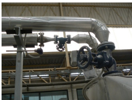
Spray dryer : Hot water control
