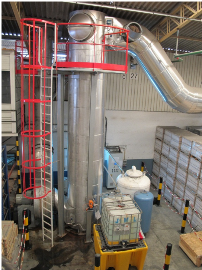
Luwa Air-Water Heat Exchanger : Hot water (140°C) is pumped in circulation to various Water-Air Heat exchangers at energy consumers (e.g. Spray dryer, Dryers)
